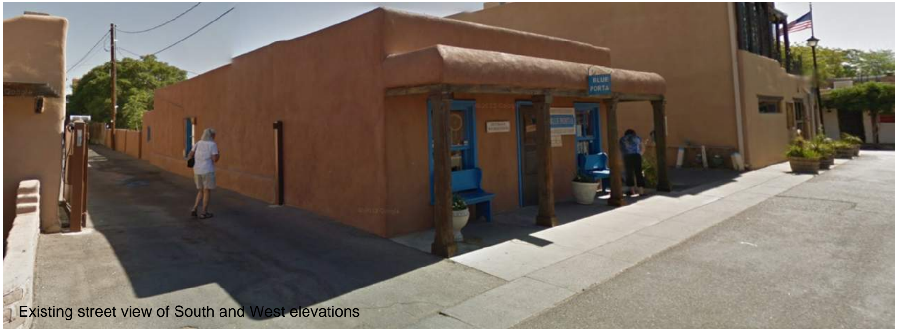
Existing street view of South & East elevations
