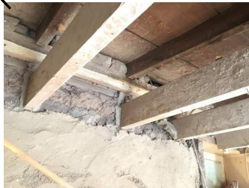
2x4 wood joist bearing at Terrone wall
